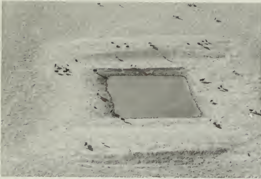
Figure 2. An example of a pit reservoir.
